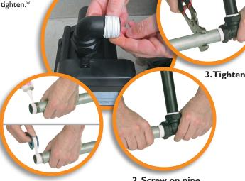
I. Apply Thread Sealant or Thread Tape
